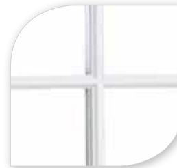
Astragal bars (applied to external glass surface)
